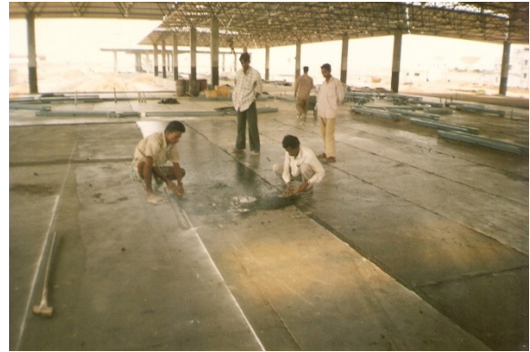
35mm thick Mastic Flooring in LPG Bottling Plant
