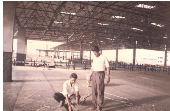
35mm thick Mastic Flooring in LPG Bottling Plant
